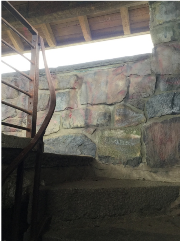
Stair E: Top of interior tower stairs, showing irregular tread depth
