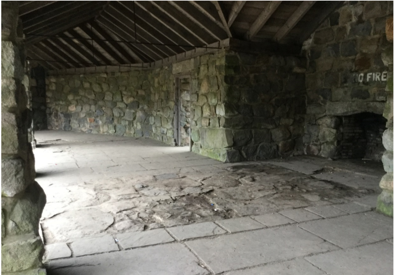
4. Interior view of pavilion showing uneven stones at fireplace hearth and surrounding flagstone flooring.
