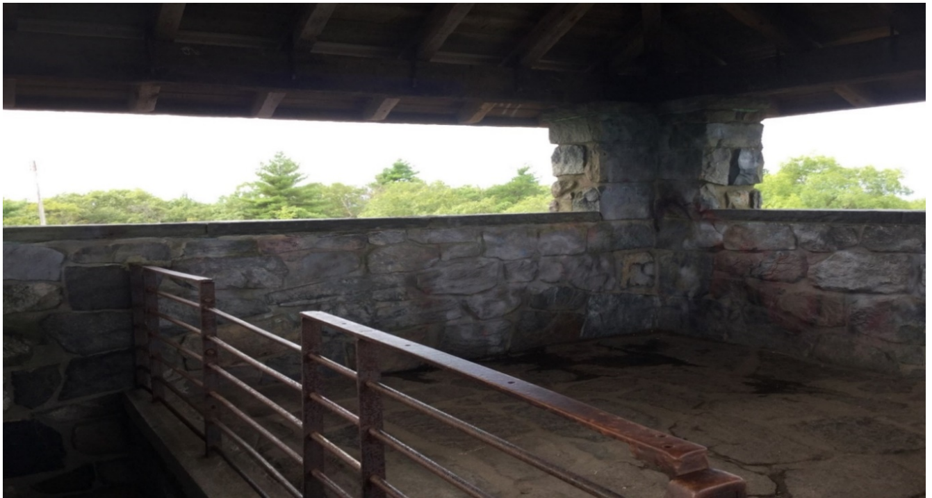
2. View of observation level from the top of the staircase, showing two of the viewing windows. Left is the West view, right is the North view. The existing railing shown will be replaced with a compliant safety railing.
