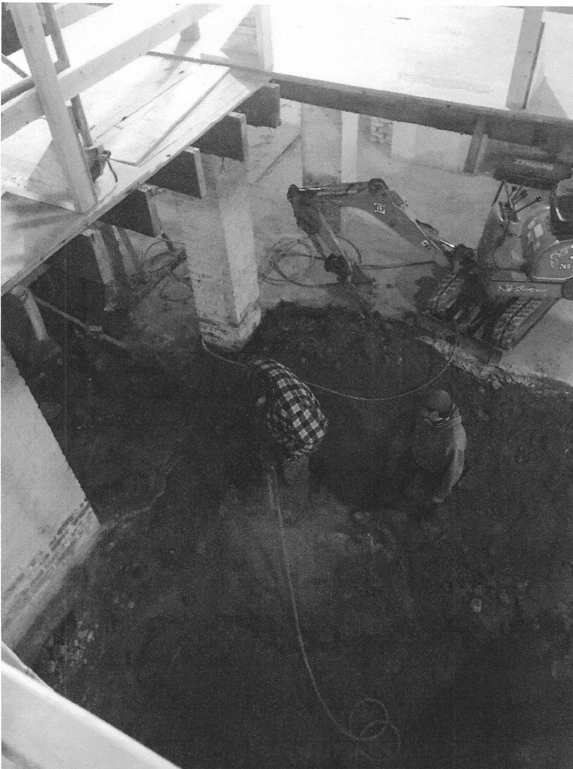
CREW JACKHAMMERING GRANITE BOULDER IN BASEMENT FOR ELEVATOR PIT NOTE MASONRY STRUCTURE AROUND PIT – DOES NOT ALLOW RELOCATION OF ELEVATOR
