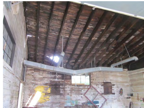
Figure 10&11: Equipment Garages & Parks Department: Completely failure of roof systems on (3) buildings
