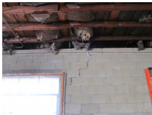
Figure 17: Failure of masonry wall at window opening
