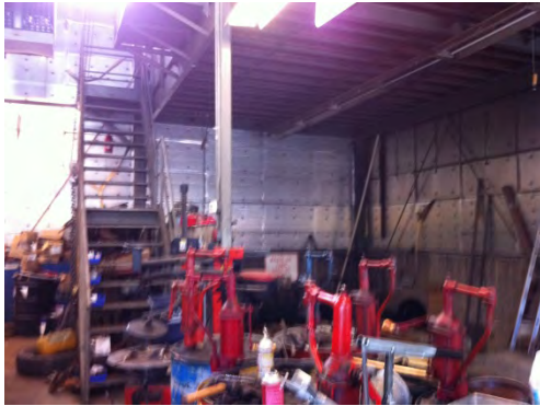
Figure 20: Non-compliant, unsafe, stairs to mezzanine
