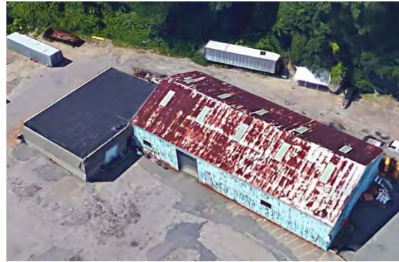
Figure 12&13: Vehicle Maintenance Ponding at Corners / Water & Sewer Department highly rusted roof
