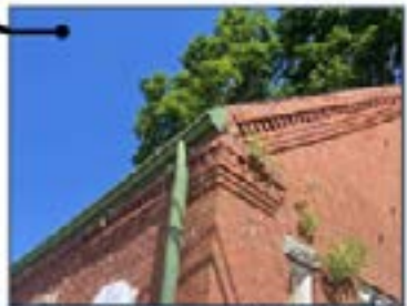
Metal Flashing and Brick Corbel
