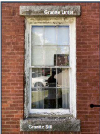
Wood Window & Granite Sill/Lintel
