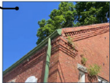
Metal Flashing and Brick Corbel
