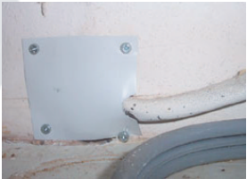
Gap sealed with metal plate
