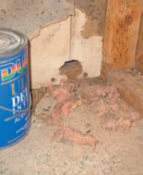
The holes that rats chew in walls tend to be the size of a tennis ball (about 2" to 3" diameter)
