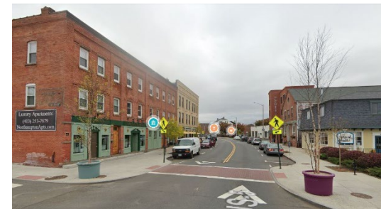
Example of curb extensions and a raised crosswalk in Northampton MA. The crosswalk is surfaced with colored and textured pavement. City snowplows are able to negotiate the curb extension and raised crosswalk without issues.
