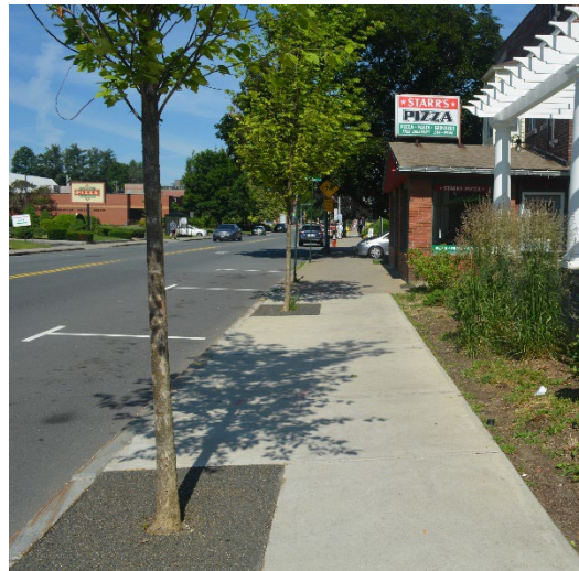
Figure 89. Tree pits can be surfaced with permeable materials, in this case permeable rubber, to allow water and air to reach plant roots, while still providing an accessible surface for pedestrians (Dodson & Flinker)
