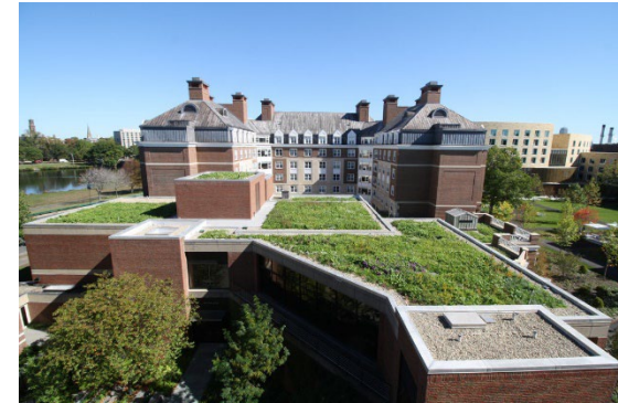
Figure 118. Green roofs can help cool buildings while absorbing stormwater and carbon (recovergreenroofs.com)
