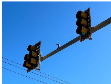
Pictured: Emergency Preemption System (Opticom) at Reed Street and Access Road intersection.
